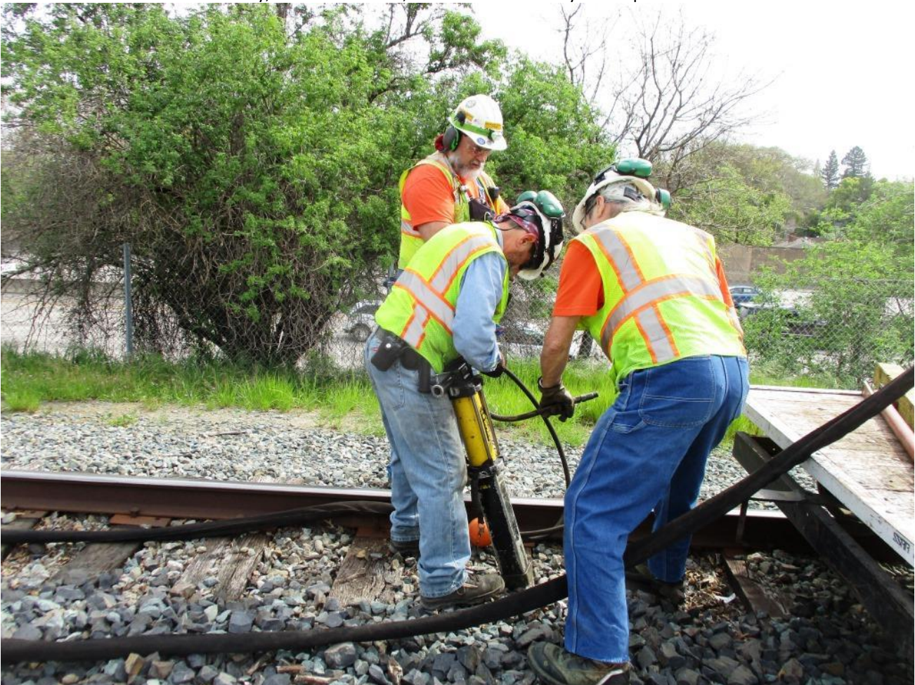
Mike F., Joe, and Ed attempt to set up the hydraulic spike puller but, soon discover, something's not quite right
