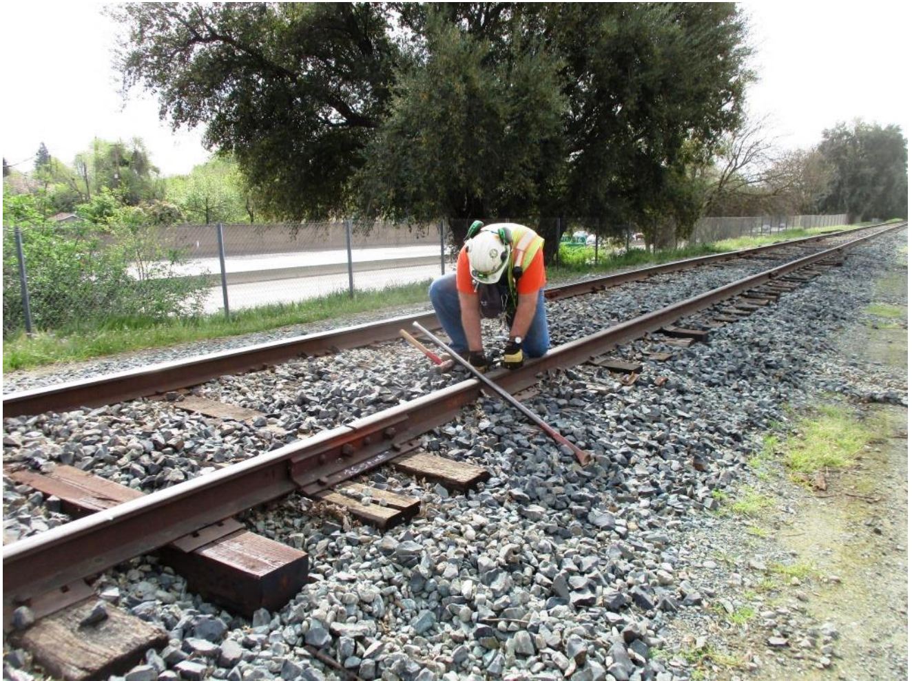
So, Mike F. resorts to pulling spikes by hand (some of which could be taken out with bare hands)
