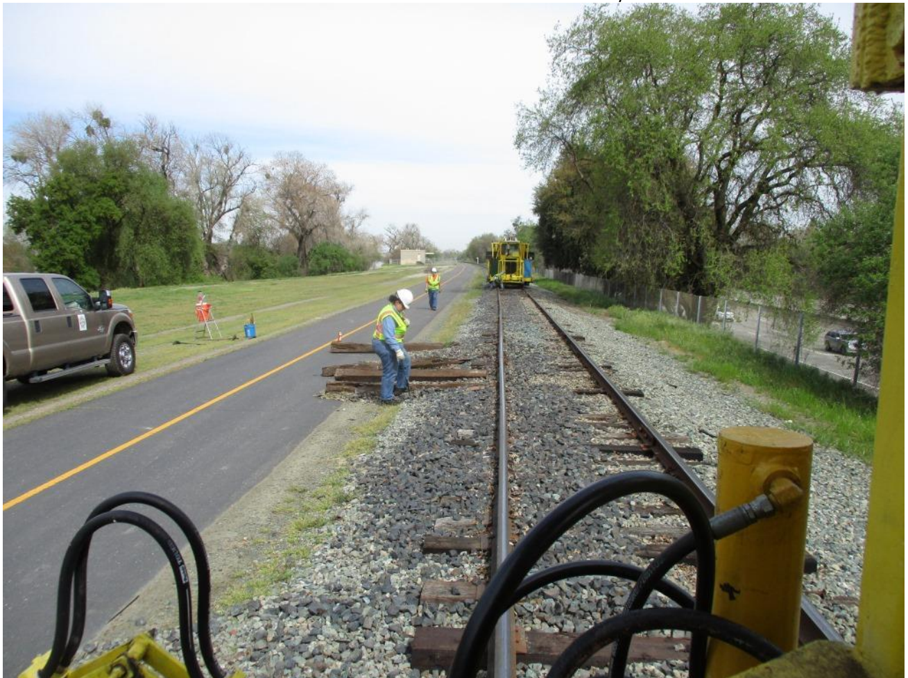
Heather lines up dead-ties for GM2 to pick up
