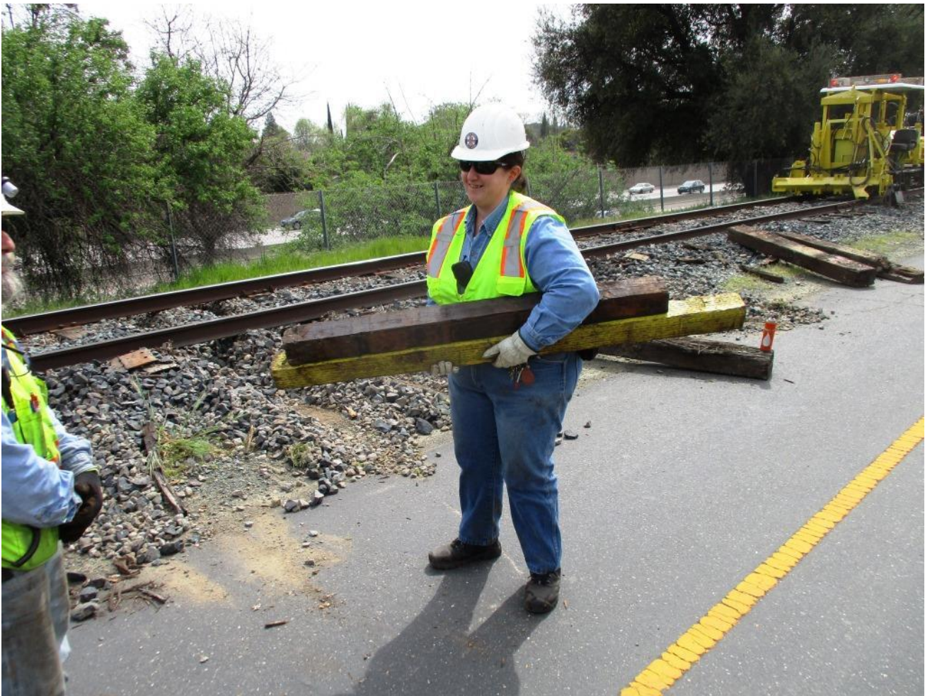
Heather carries the cribbing onto which the dead-ties can be stacked once collected
