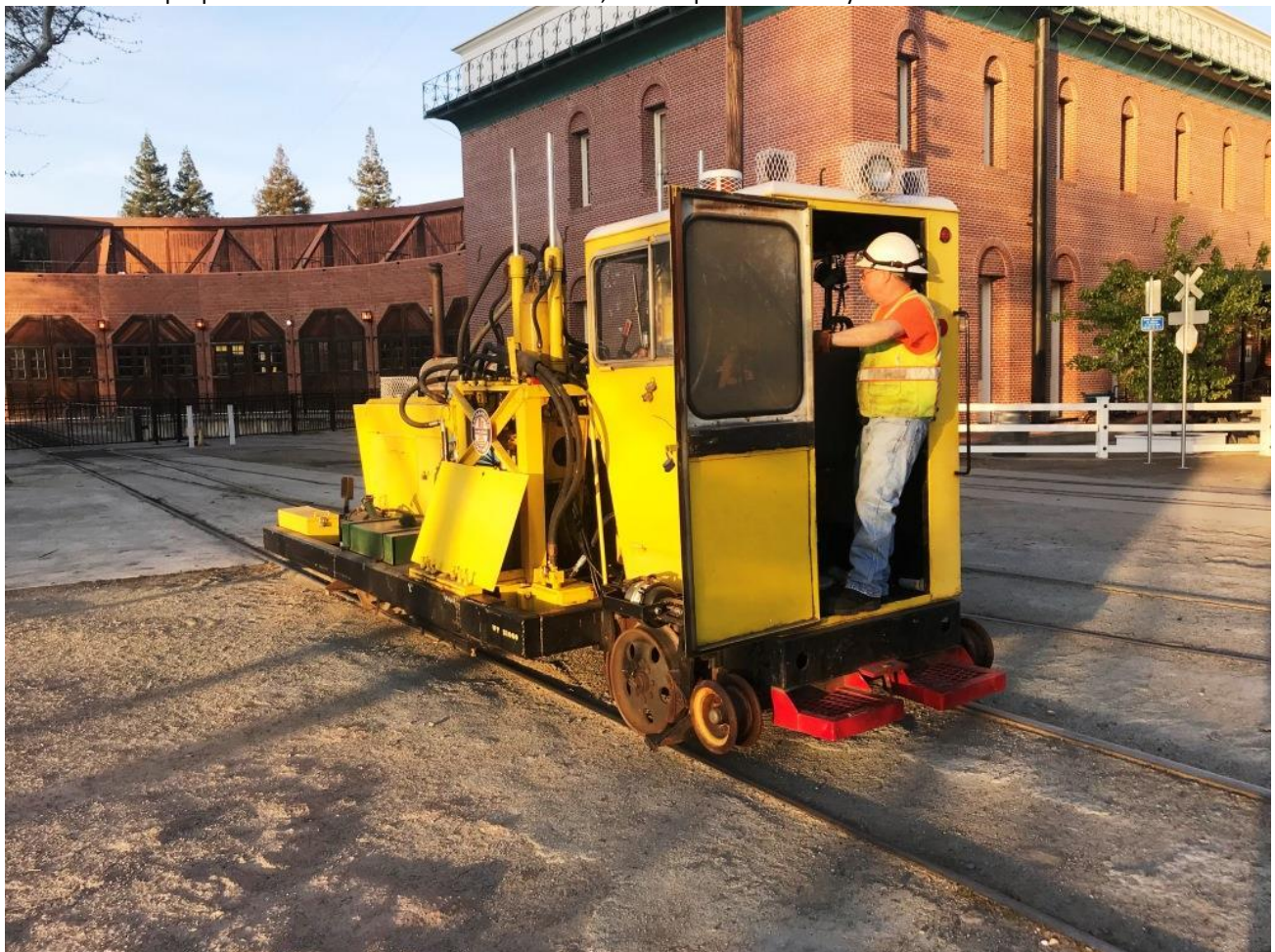
Mike H. switches out the tie-sher
