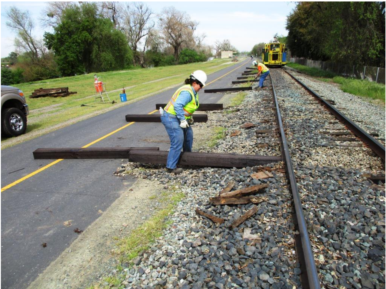
Heather gets ties line up for the Jackson 125 to insert
