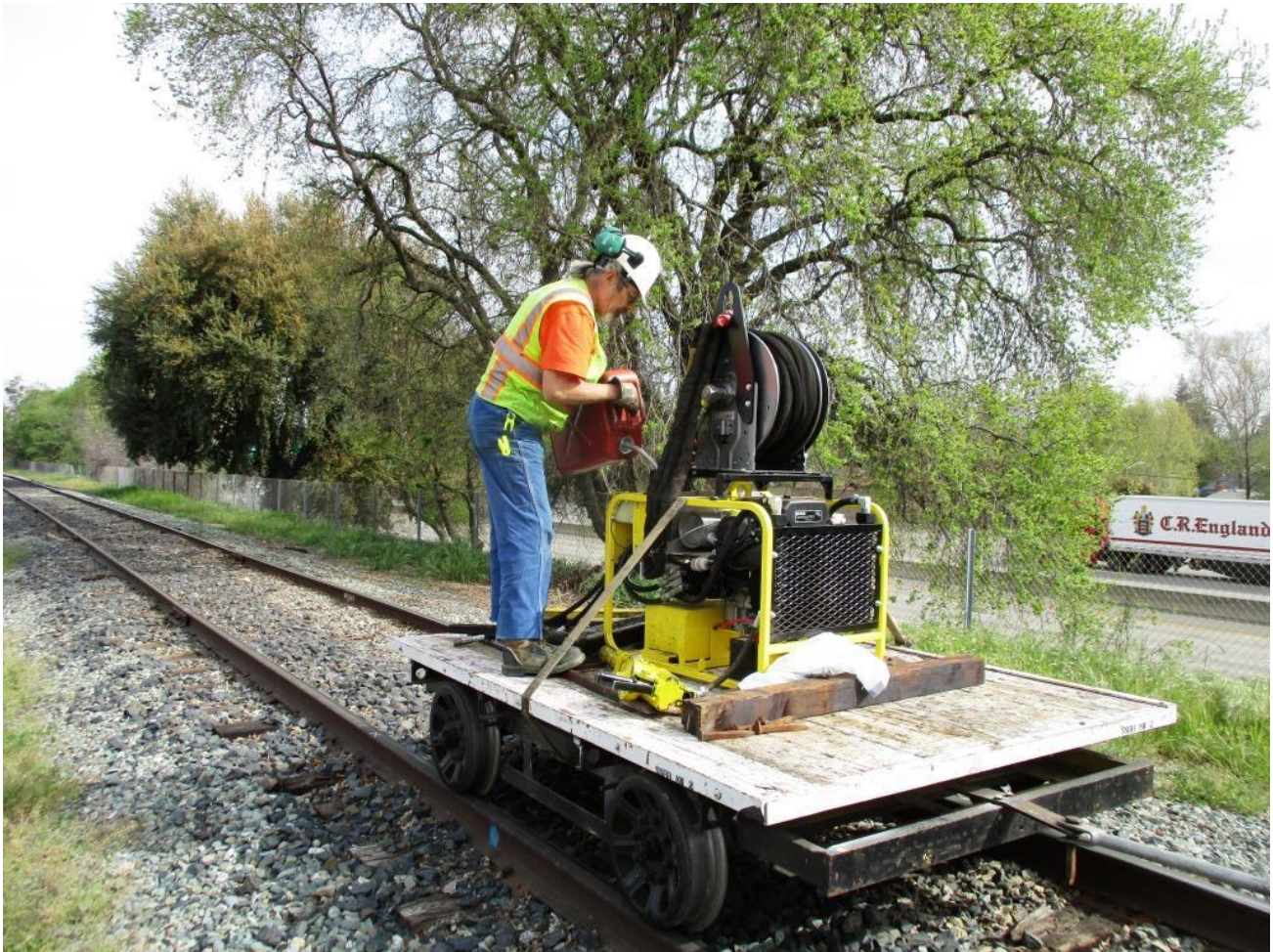
Saturday, down on the line, Ed adds fuel to the hydraulic power unit
