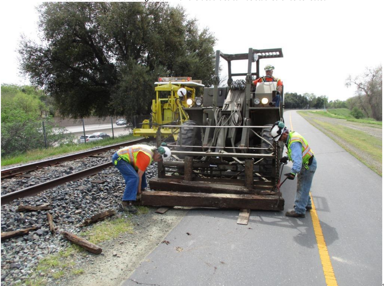
Ed and Joe slide dead-ties onto the forks of GM2
