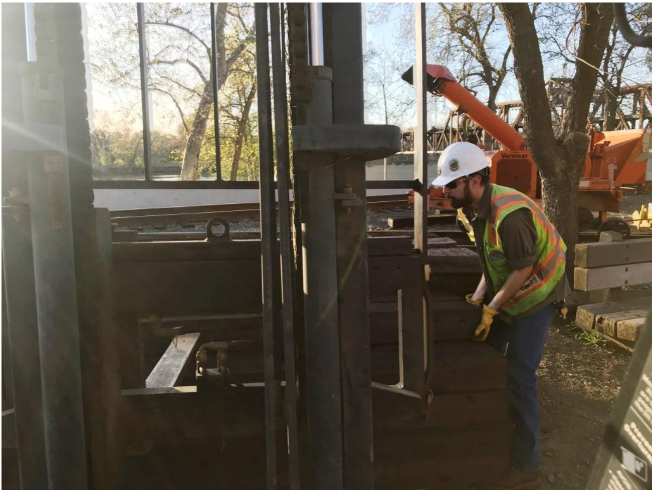
As the propane forklift moves ties off the flatcar, Matt repositions a wayward tie that started to roll-off
