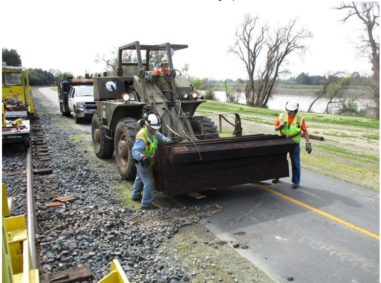
Joe and Ed deploy new ties at each empty tie-crib
